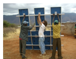
solar panels at Mforo
