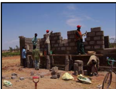
Construction of Teacher Housing at Secondary School
