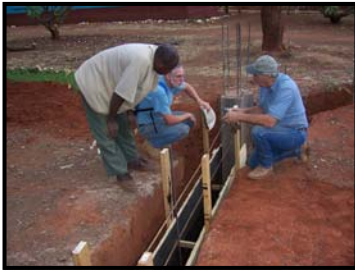
Foundation Construction of the Chapel
